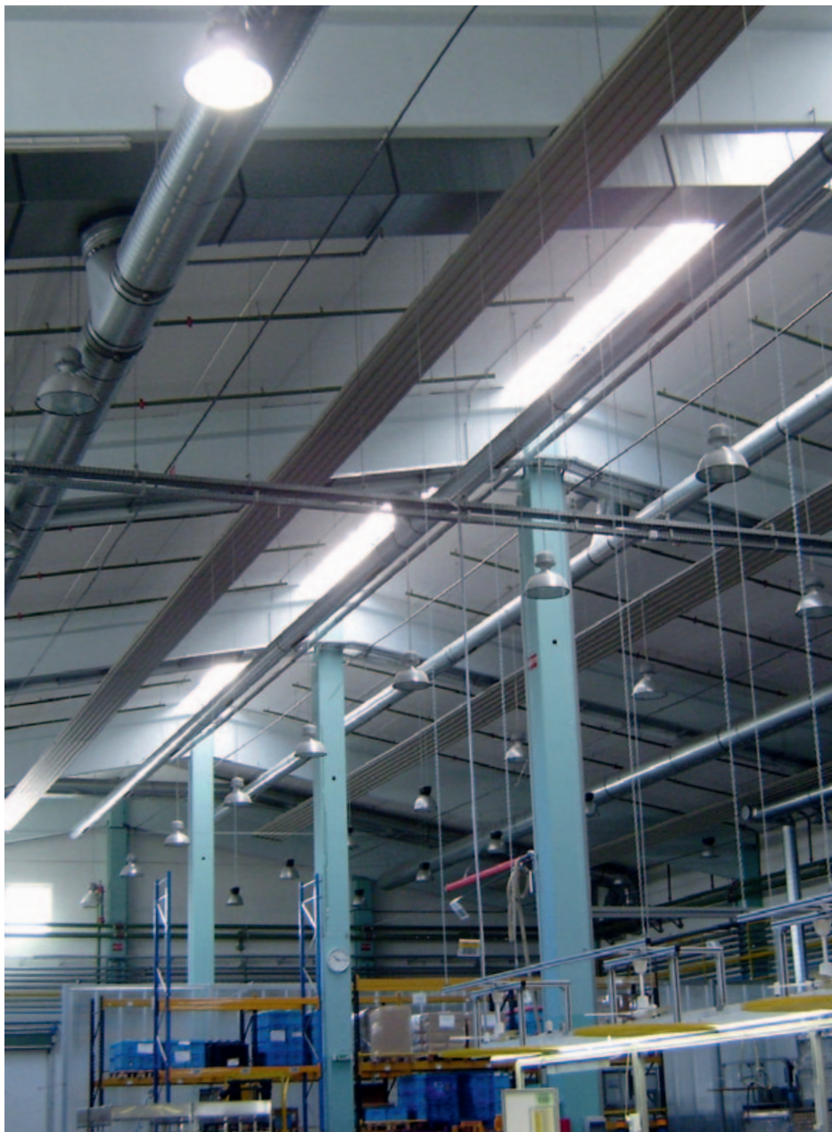
At the St. Michael plant, an energy team has been appointed to formulate and implement improvements and savings in all areas relating to energy and the environment. For example, targeted workplace lighting has reduced the continuous load of the factory lighting, and additional energy has been saved through the use of low-power lamps.
